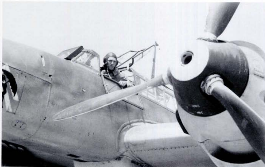
LEFT: An unknown pilot of 7./ZG 26 prepares for a mission. Note the 7. Staffel emblem on the nose, the armoured windscreen, spinner tip in the Staffel colour of white and the angle of dive line on the lowered pilot's window.
