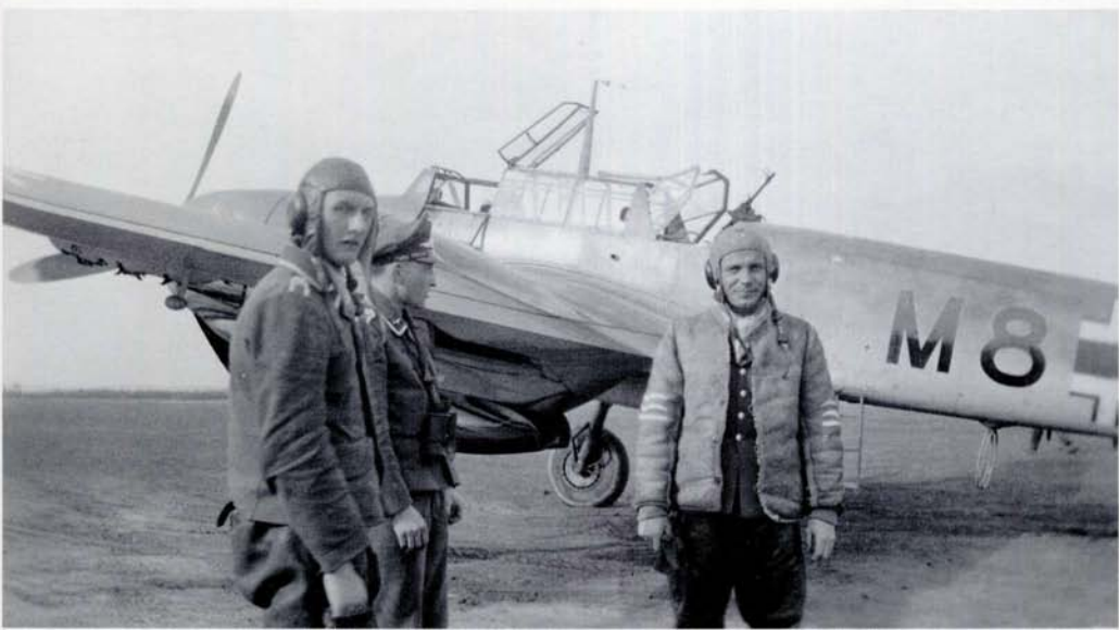
LEFT: An unknown Oberleutnant poses with two Unteroffiziere in front of a Bf 110 of II./ZG 76 . The cable along the top of the fuselage and the under wing bomb rack identify the aircraft as an 'E' variant. Note the 'N' on the port engine cowl, denoting the fitment of the DB 601 N engine. Heavy staining can be seen on the port undercarriage door.
