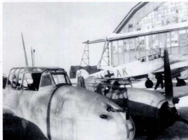
BELOW: 3U+AK of 2./ZG 26 during the winter of 1941/42 on the Russian Front. Note that unlike the Bf 110 of (F)/Aufkl. Gr. 33 in a previous photograph, this Bf 110 has its canopy framing painted white as well as the main areas of the aircraft.
