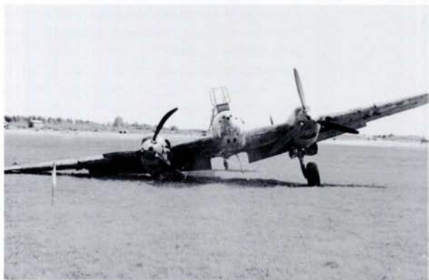
BELOW AND BOTTOM: Two views of a Bf 110 E belonging to the Gruppenstab of I/SG 1 that has suffered a collapsed starboard undercarriage.
